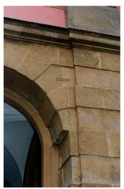
In 2002 - conservation of stonework on the front elevation, works embraced stoneworks of cornice, window frames, plinths and galleries as well as stucco.
